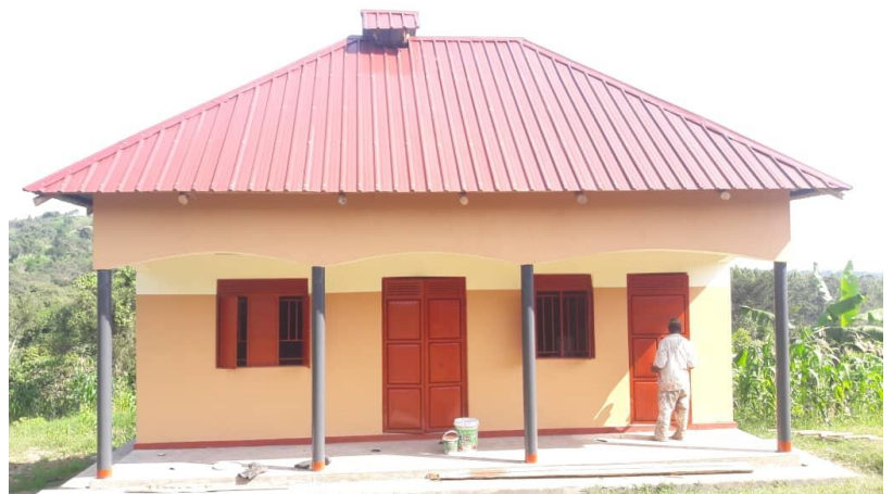
New kitchen (big door is the main Kitchen, small door is store & cook theaster/changing room)
